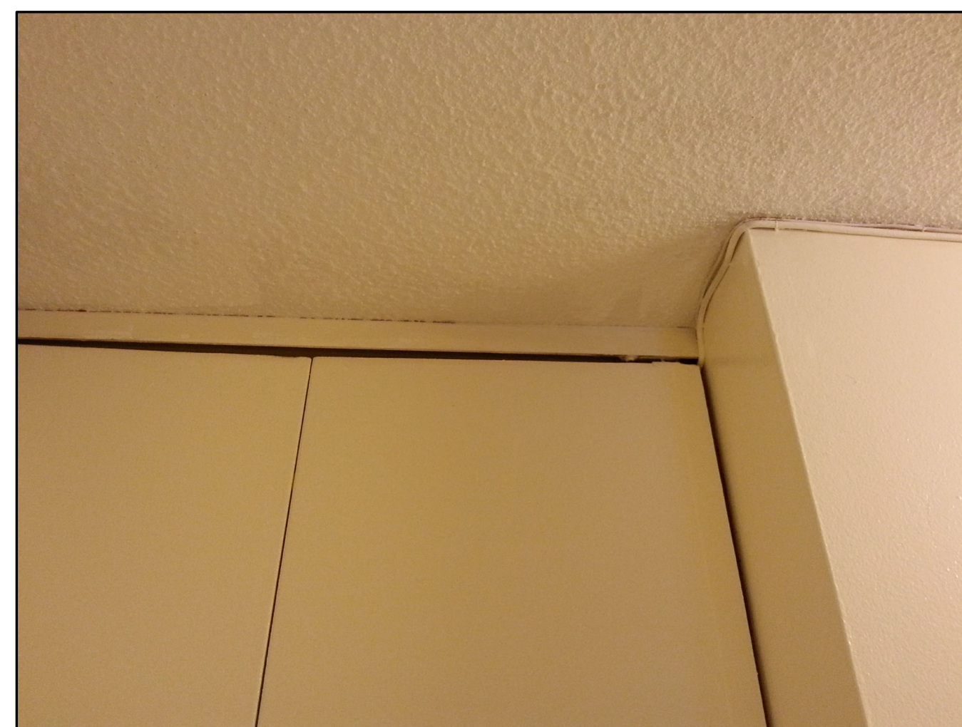
NOTE: CONTRACTOR TO COORDINATE WITH FIT PRIOR TO DEMOLITION OF EXISTING TRACK.
