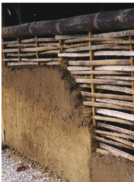
Figure 1. Sustainable building structure utilizing dried bamboo strips and adobe.
